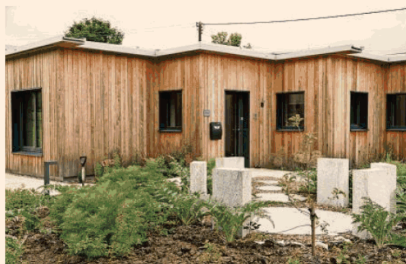
Larch Corner, designed by LEAP – Mark Sidall
